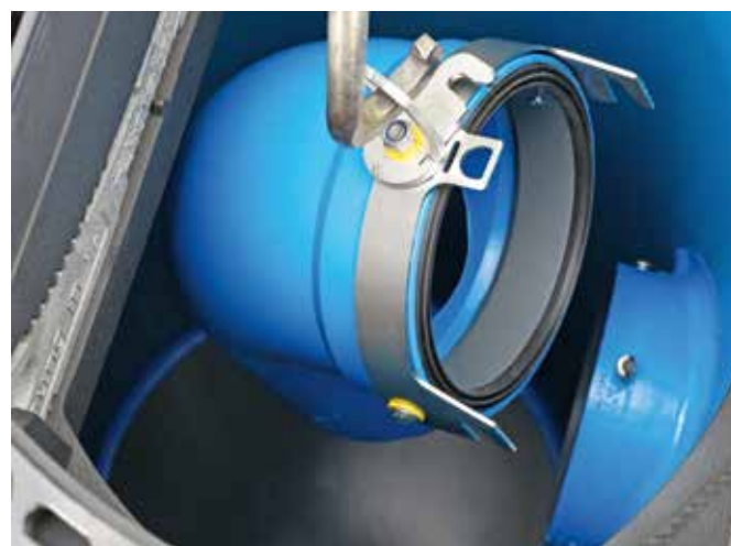
The locking tab is rotated by at least 45° and the built-in part can then be removed
