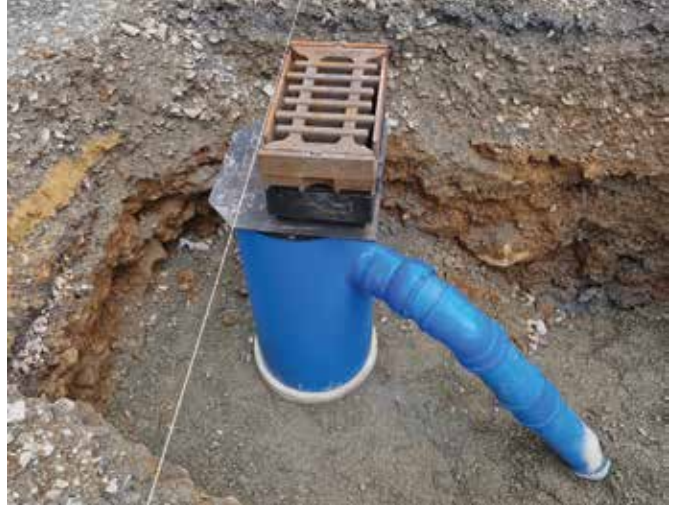
The support jaws and bushes allow perfect adjustment of the height and tilt level
