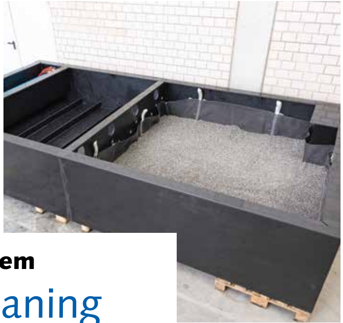
Installing the Funke Area-Clean-substrate
