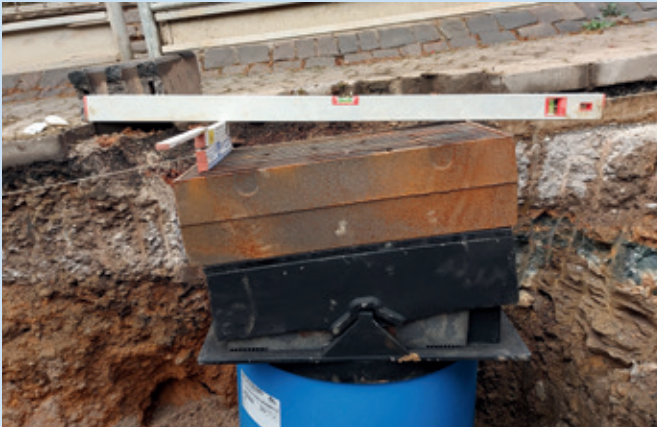
Thanks to the support jaws and bushes, the required height and gradient can be perfectly adjusted.
