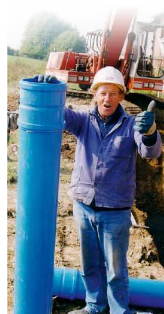
One of the first schemes with HS®-Underground Drainage Pipes went swimmingly
