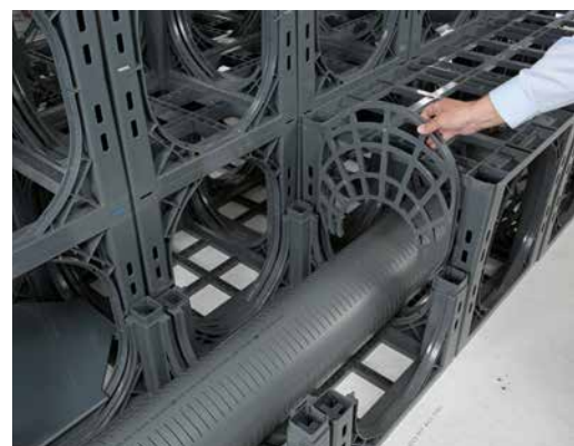
Installing the jetting pipe
