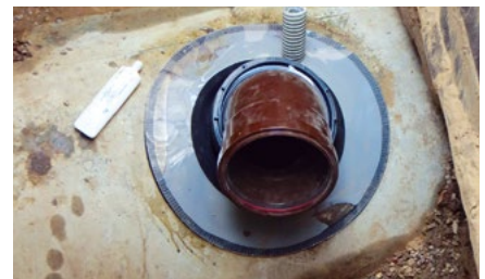
A special casting resin ensures a water-tight connection.
