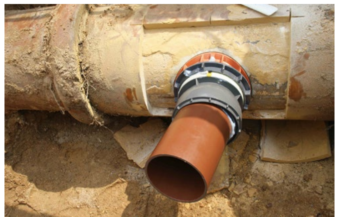
Installing the CONNEX Liner Connection System: The sealing compound is introduced through an opening in the spacer ring.
