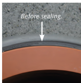
Junction is in the right position but not compressed.
