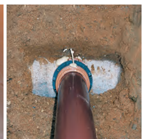
Junction is installed in a concrete pipe connecting a DN 160 mm diameter HS-Pipe carrying waste water.
