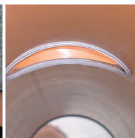
Correct installation of the junction.
