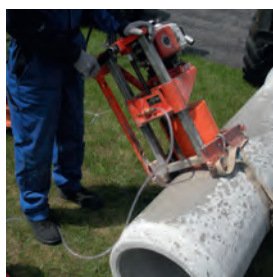
Correct Coredrilling
